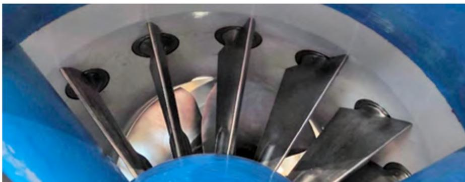
an elastic coupling. As a part of the overhaul there has been an appraisal and a repair of the entire hydraulic profiling of the turbine (including: its intake, guide vanes, turbine's cover, runner, runner's chamber, and turbine's suction pipe). Moreover, among other things – all the sealings and bearings have been replaced, together with the shaft connecting the runner to the generator. Faro Quantum ScanArm 3D scanning device has been utilised during the appraisal and repair of the profiling.
