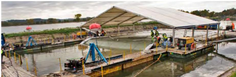
Fig. 8. Canal de Jonage, Installation of Incomat® Standard panel from a pontoon, together with the application of anchor loops to piles to stabilise the mats in flowing water conditions 1994, photo: Huesker.
